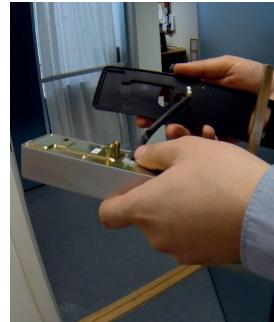
A 2 mm extension bracket is also included, which must be used if the distance between the lock case and the bolt becomes too large, so that the lock box's hook bolt does not automatically fold out when the door is closed.
