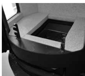
Place front and rear base brick Front front brick has a chamfer which faces towards door glass.
