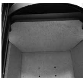
Baffle in position resting on supports.
