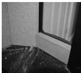
Place front side bricks into position, place side brick into groove at front edge of the stove.
