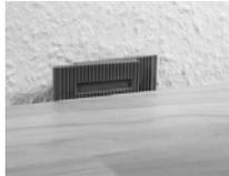
3. Use the spacer wedges to guarantee the expansion space of at least 8 - 10mm towards all walls and structural parts within the room.
