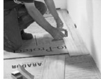
2. Center and align the planking area and cut the first row to size.
