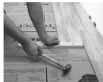
6. Join the short end sides together using a hammering block. Continue to install the rest of the room in this manner. (Laminate Flooring Trendtime 1 and 2 are featuring a different type of locking mechanism on the shortend side. Details on page 13.)
