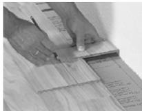
7. Use a cut-off piece to transfer the profile of the wall to the last row of planks.
