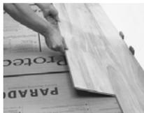
5. Start your next row from the left hand side like before. Simply click together the planks' longitudinal sides. The use of glue is not required here.
