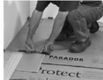
4. The last board of the first row is cut to the right size - don't forget to include the wall spacing. The cut-off piece is used as the starting piece for the second row.
