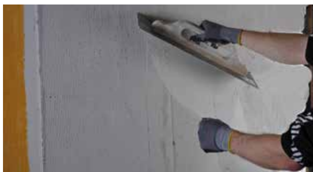
Montering af net med min. 10 cm overlap
