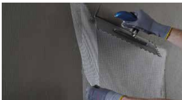
Montering af net med min. 10 cm overlap
