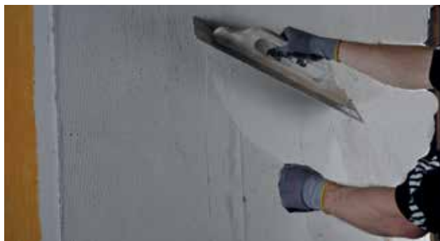
Montering af net med min. 10 cm overlap
