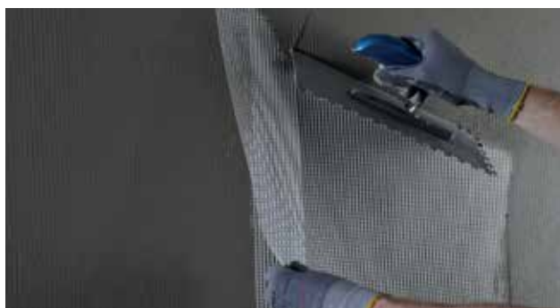
Montering af net med min. 10 cm overlap
