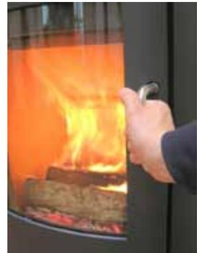
8. Reduce the amount of combustion air to the desired position, and optimal combustion will continue until there are glowing embers in the bed.
