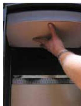
6. Make sure that the baffles and brick panels are correctly assembled before lighting the stove after cleaning.
